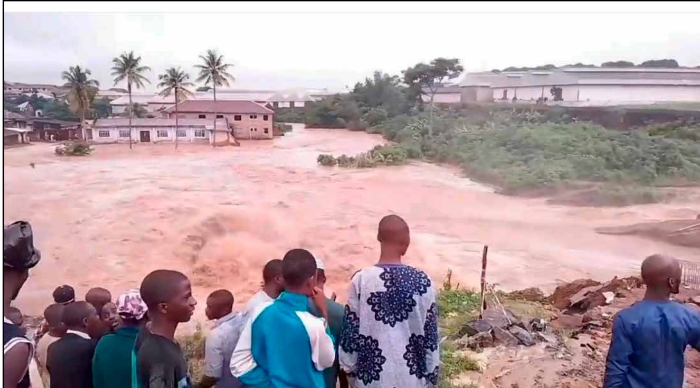
Flooded Olodo Bridge-Iwo Road, Ibadan, Oyo State after the downpour...on Sunday.
